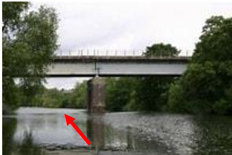
Looking downstream to the railway bridge.
